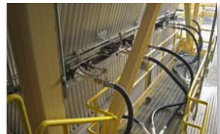
Sorbent Injection system delivers the correct combination of sorbents.
